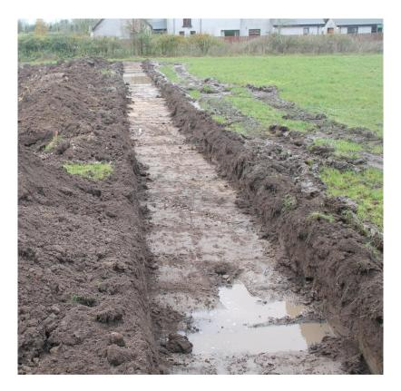
Plate 15. Ardboe, Co. Tyrone. Looking back along Long Trench 8. Stone drain with red brick cut into subsoil in foreground, two field drains running diagonally across the trench in the middle of the shot and water covering a field drain at the eastern end of the trench in the background. From the east.
